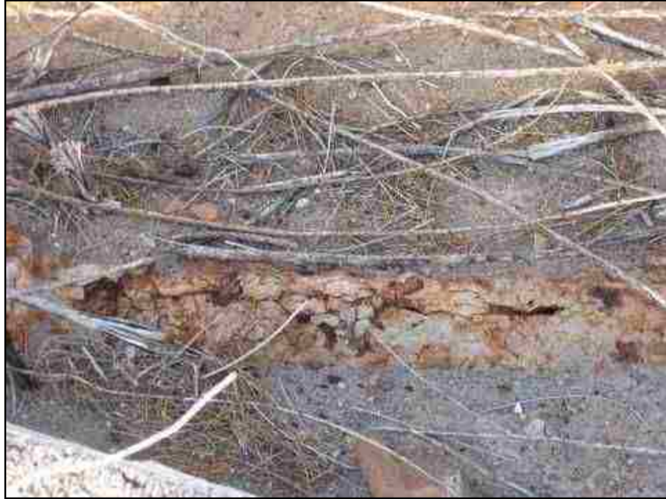
Figure 27: Possible sewer pipe at the Gentry Hotel, February 2008. Photo by author.
