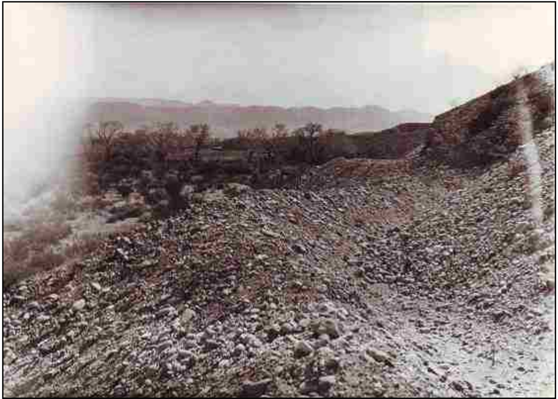
Figure 10: Pioneer irrigating ditch in the Moapa Valley. Courtesy Boulder City Museum.
