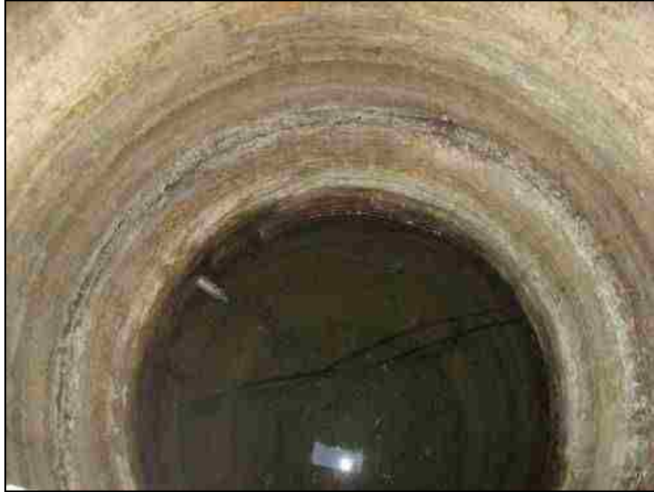
Figure 25: Post office cistern, February 2008. Photo by author.
