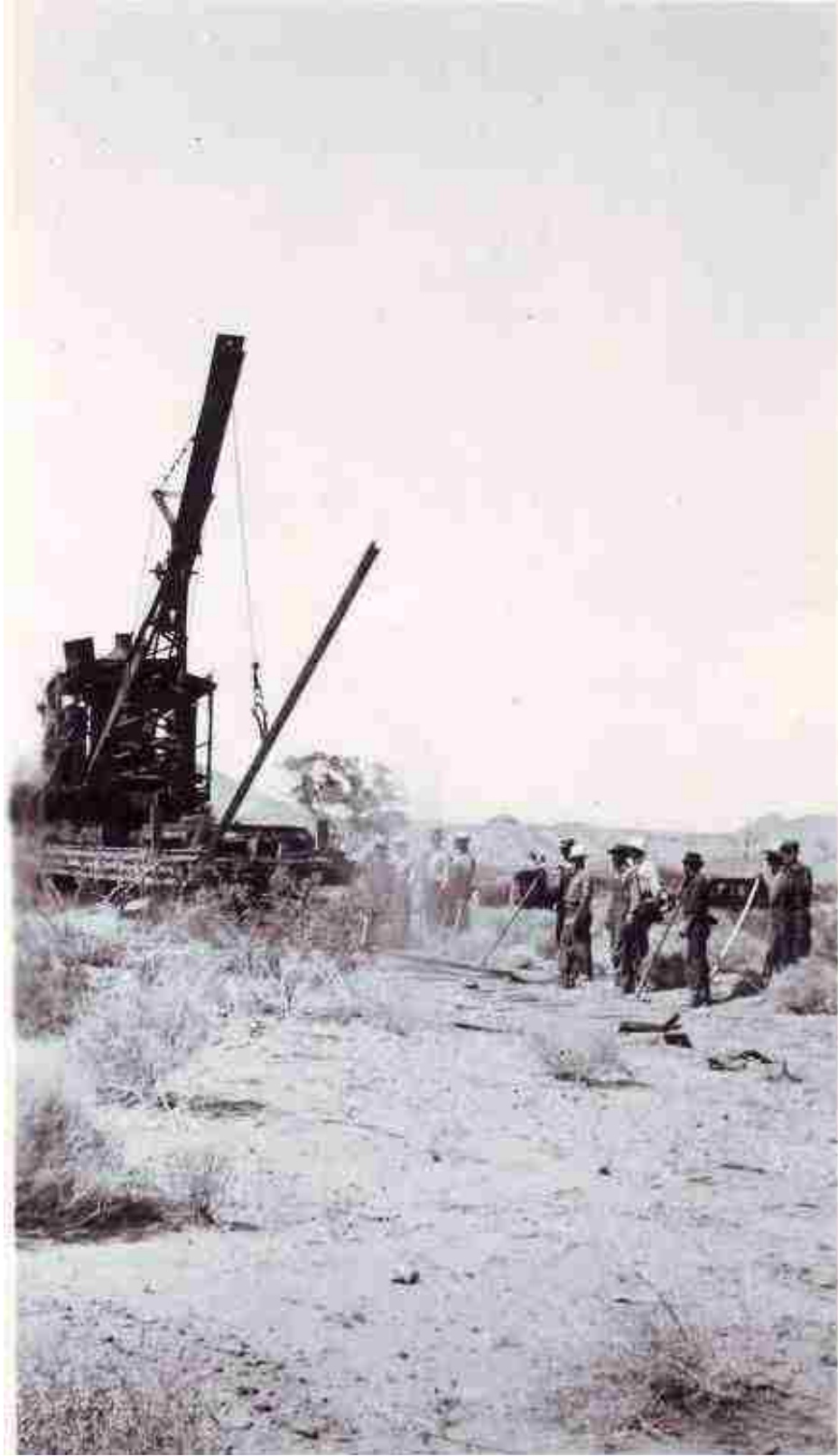
Figure 42: Union Pacific Railroad crew dismantling rails near St. Thomas. Courtesy Boulder City Museum.
