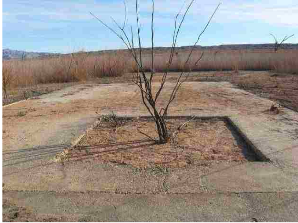
Figure 13: Foundations of Hugh Lord's garage. Note the tree growing in the grease pit.
