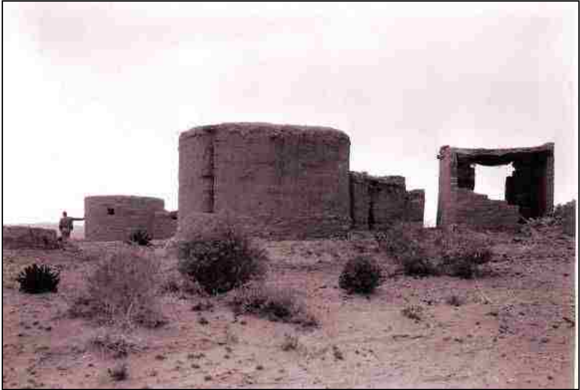
Figure 3: Lost City reconstruction, 1939. Bureau of Reclamation, Office of Chief Engineer, Boulder Canyon Project, album 7. NARA Denver.
