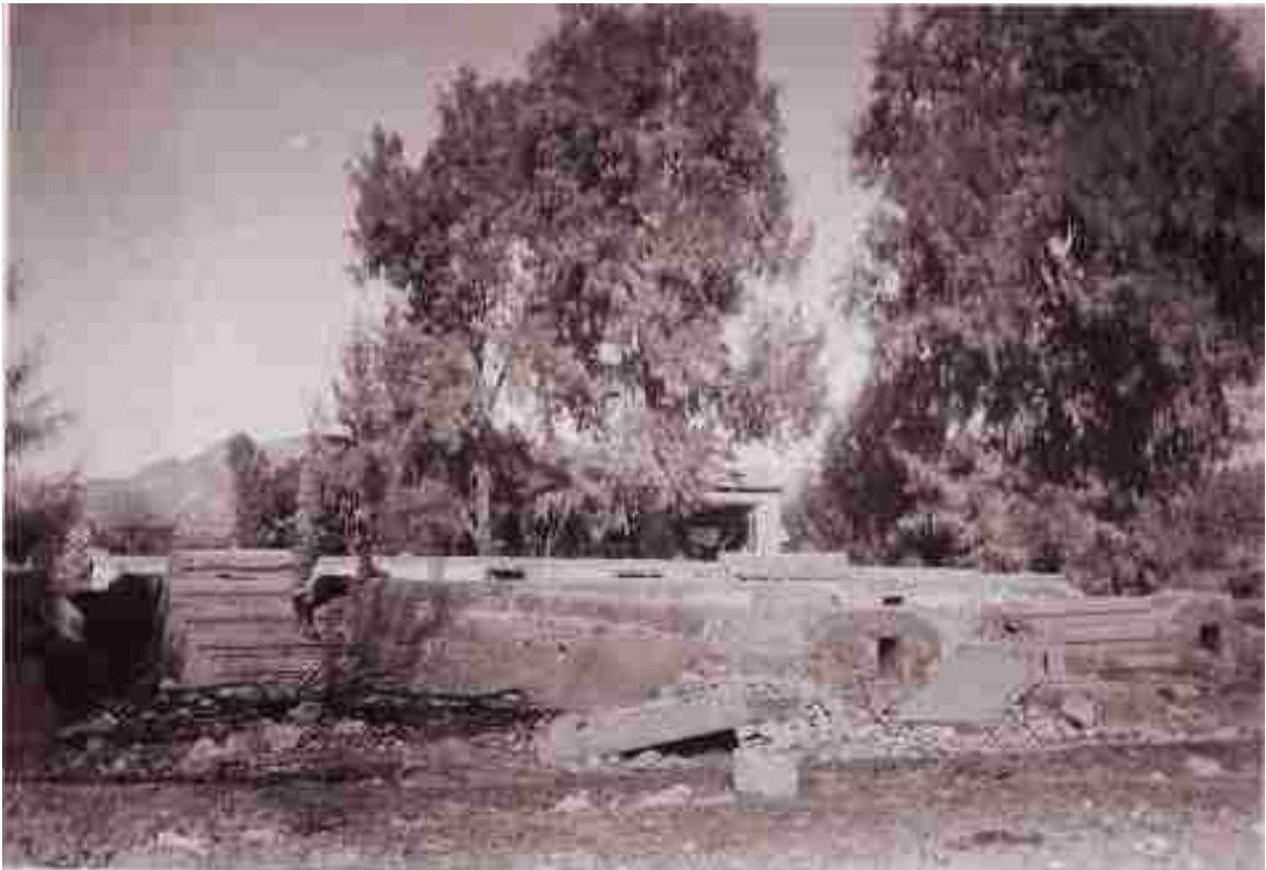
Figure 37: Abandoned foundation, 1935. Bureau of Reclamation, Office of Chief Engineer, Boulder Canyon Project, album 4. NARA Denver.
