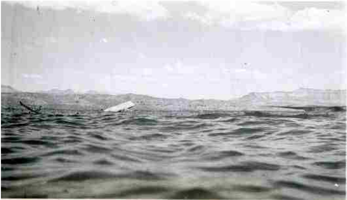
Figure 53: Foundation of the schoolhouse going under. Edwards Collection, UNLV Special Collections.
