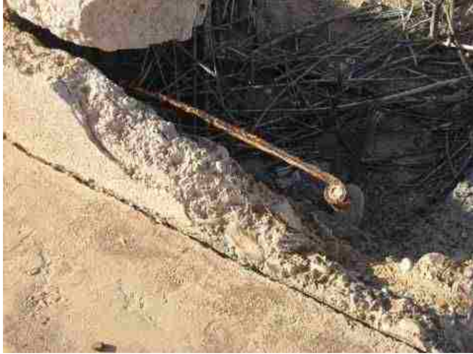
Figure 29: Automobile spring reinforcing the concrete in Hannig's Ice Cream Parlor.
