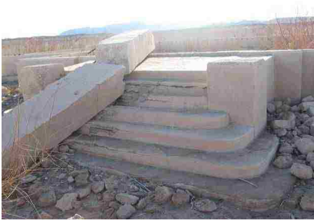
Figure 17: Steps of the schoolhouse.
