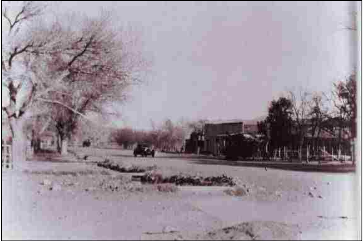
Figure 28: Automobile in St. Thomas. Courtesy Boulder City Museum. Harry Gentry's store is on the right. In the foreground is the only concrete conduit/bridge in the town.
